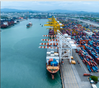
Ports energy backup
