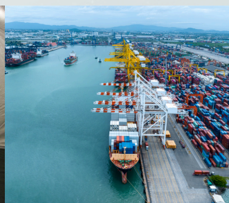
Ports energy backup
